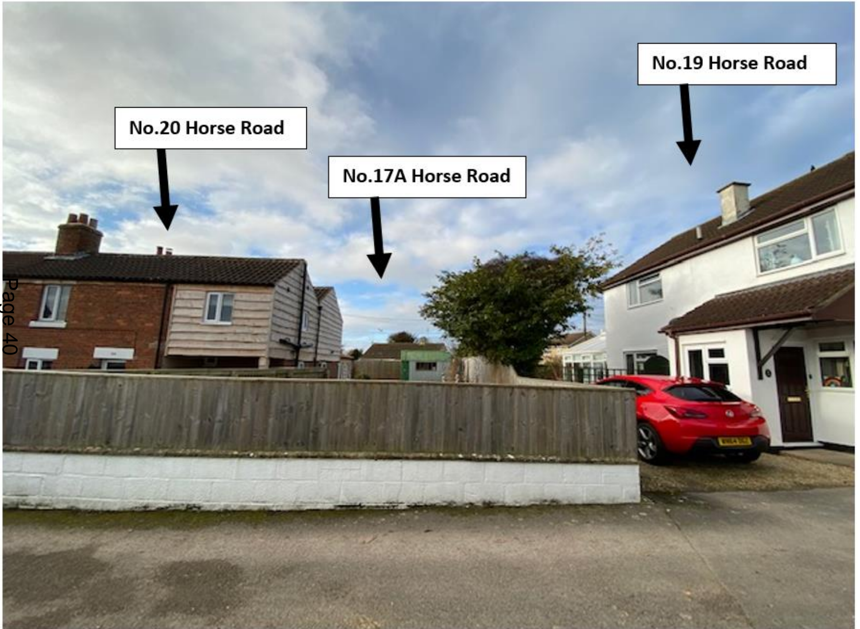
View of site from No.20 and No.19 Horse Road access lane
