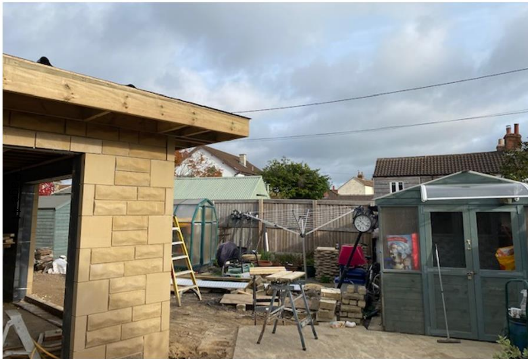
View of from No.20 and No.19 Horse Road from site
